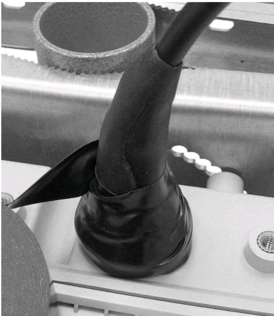
8. Continue wrapping the vinyl electrical tape in a spiral back down to the filter. You should now have two layers of vinyl electrical tape covering the Butyl rubber.
