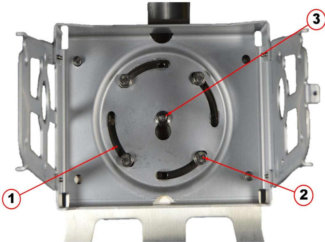
6. Insert the four (8mm x 25mm) mounting screws supplied with the installation kit into the threaded holes in the base mounting plate. Do not tighten bolts until all are started.
