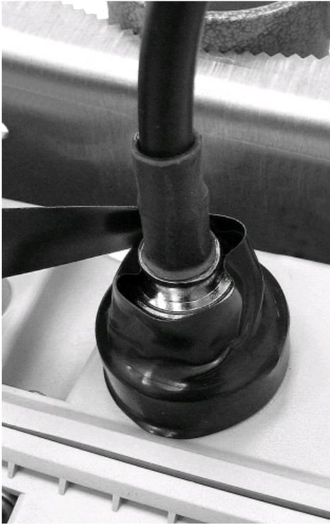
The vinyl electrical tape provides a foundation for the Butyl rubber sealant, making it easier to disconnect the cable.
