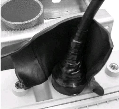
5. Ensure that the Butyl rubber extends past the vinyl electrical tape and onto the cable jacket.
